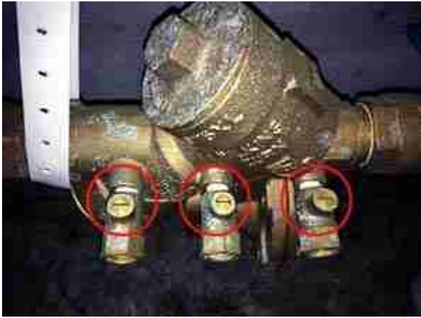
Fig. 4 Petcock Valves should be in CLOSED position (perpendicular to pipe)
