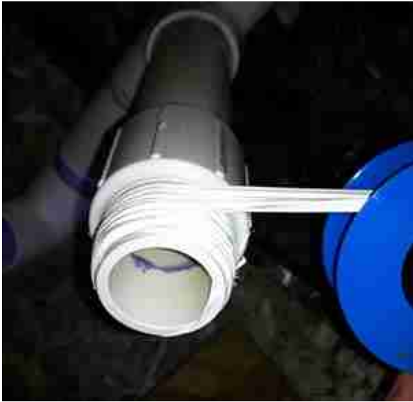
Fig. 2 Wrap Teflon Tape before replacing cap
